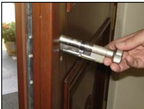
Rotate locking strike until it is flush with the cylinder. The strike needs to be flush so you can slide it into the pre-mortised hole and interior hardware. With the door opened, slide the key cylinder into the pre-mortised hole.
