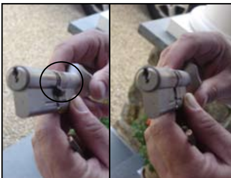
Rotate locking strike until it is flush with the cylinder. The strike needs to be flush so you can slide it into the pre-mortised hole and interior hardware. With the door opened, slide the key cylinder into the pre-mortised hole.
