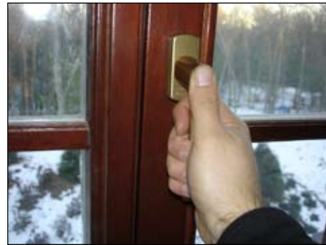
(1) With the unit fully closed and locked, loosely set the handle into place.
