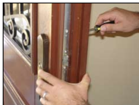
Slide the two screws into the interior escutcheon plate. Slide the screws into the pre-mortised holes until the screws make contact with the exterior plate. Gently screw by hand, then loosely tighten with screw driver .
