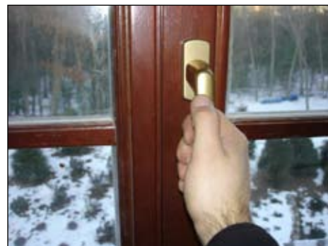
(5) Close the window sash and turn the handle down into the Closed-Position.
