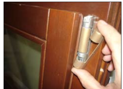
Remove top Hinge Cover
