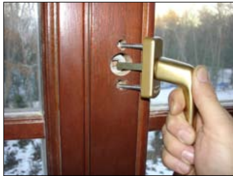
(1) With the unit fully closed and locked, loosely set the handle into place.
