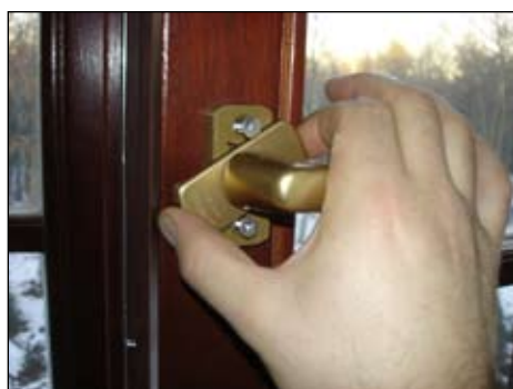
(3) Once the unit is opened and handle is horizontal, pull and rotate the hardware cover to expose the screws.
