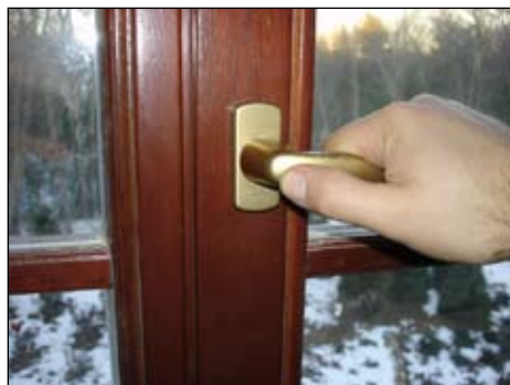
(5) Close the window sash and turn the handle down into the Closed-Position.
