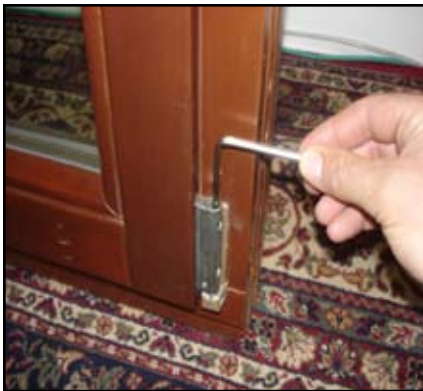
Clockwise to Raise the Sash
