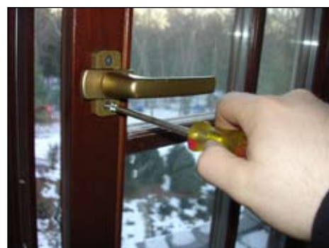
(4) Ensure both screws are accurately positioned into the mortised holes, then tighten with a Phillips screwdriver.
