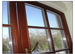
Rotate the handle approximately 135 degrees, then gently pull to micro-tilt open the sash. Always push close the sash before attempting to change the handle position.
