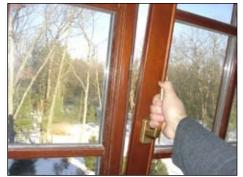
Rotate the handle up 180 degrees, then gently pull to tilt-open the sash. Always push close the sash before attempting to change the handle position.
