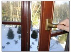
Rotated the handle horizontally, then swing open the sash.
